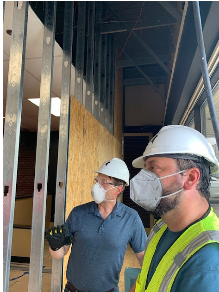
Vessko and Guy explaining about Temporary protection
