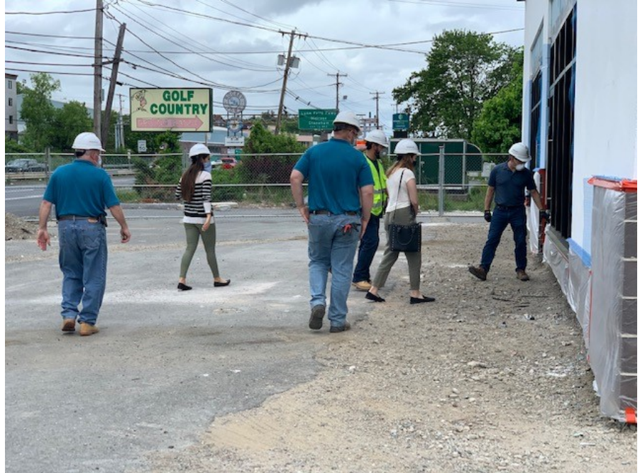
Guy explaining about the customized windows
